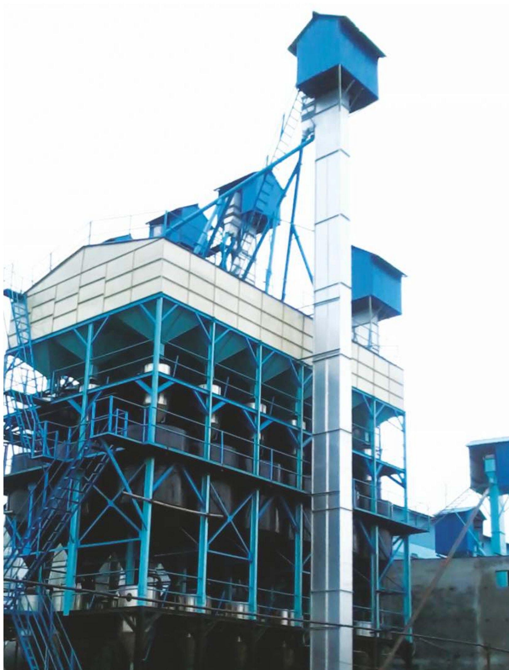
3 X 24 TON THREE STAGE PLANT
