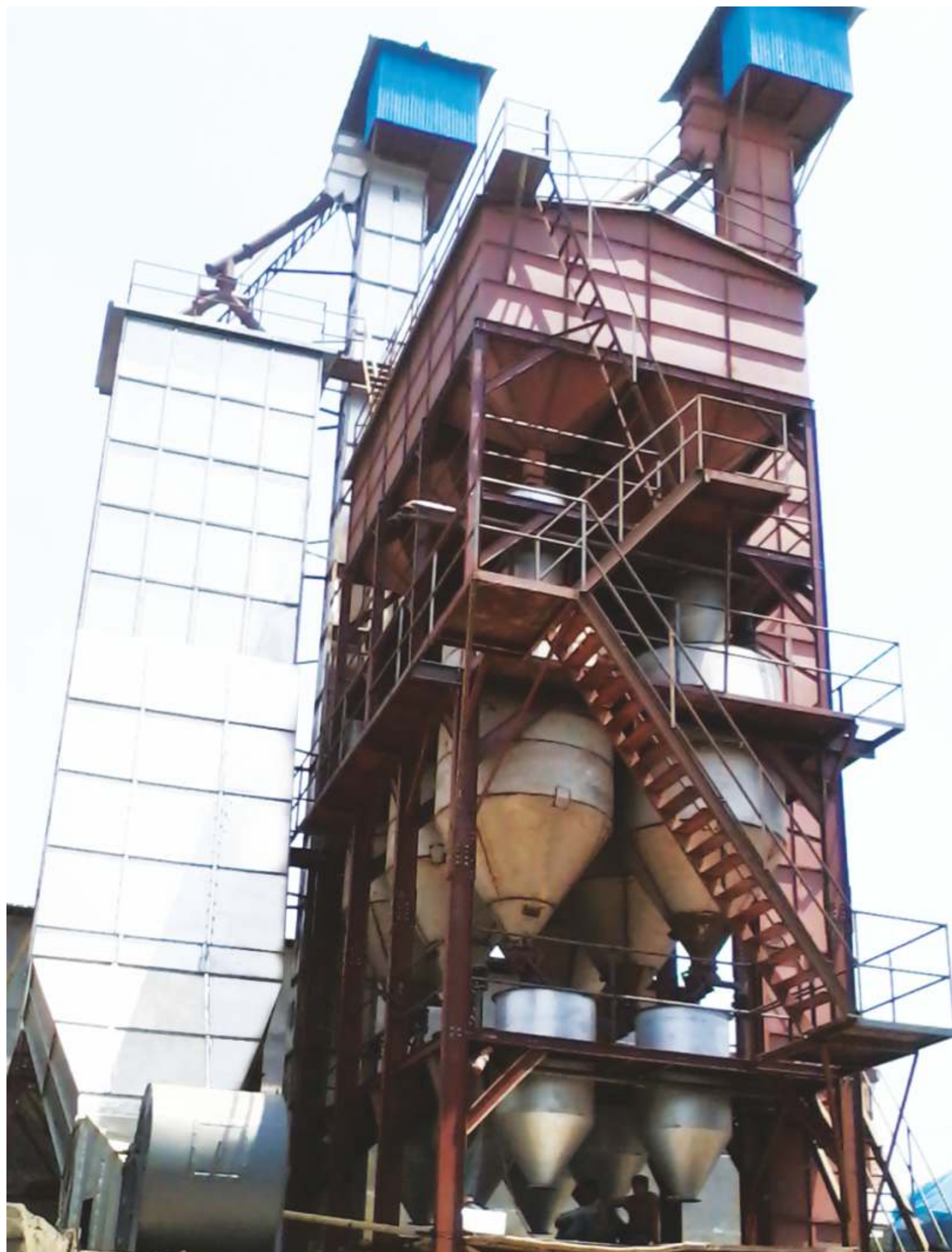
1 X 24 TON THREE STAGE PLANT
