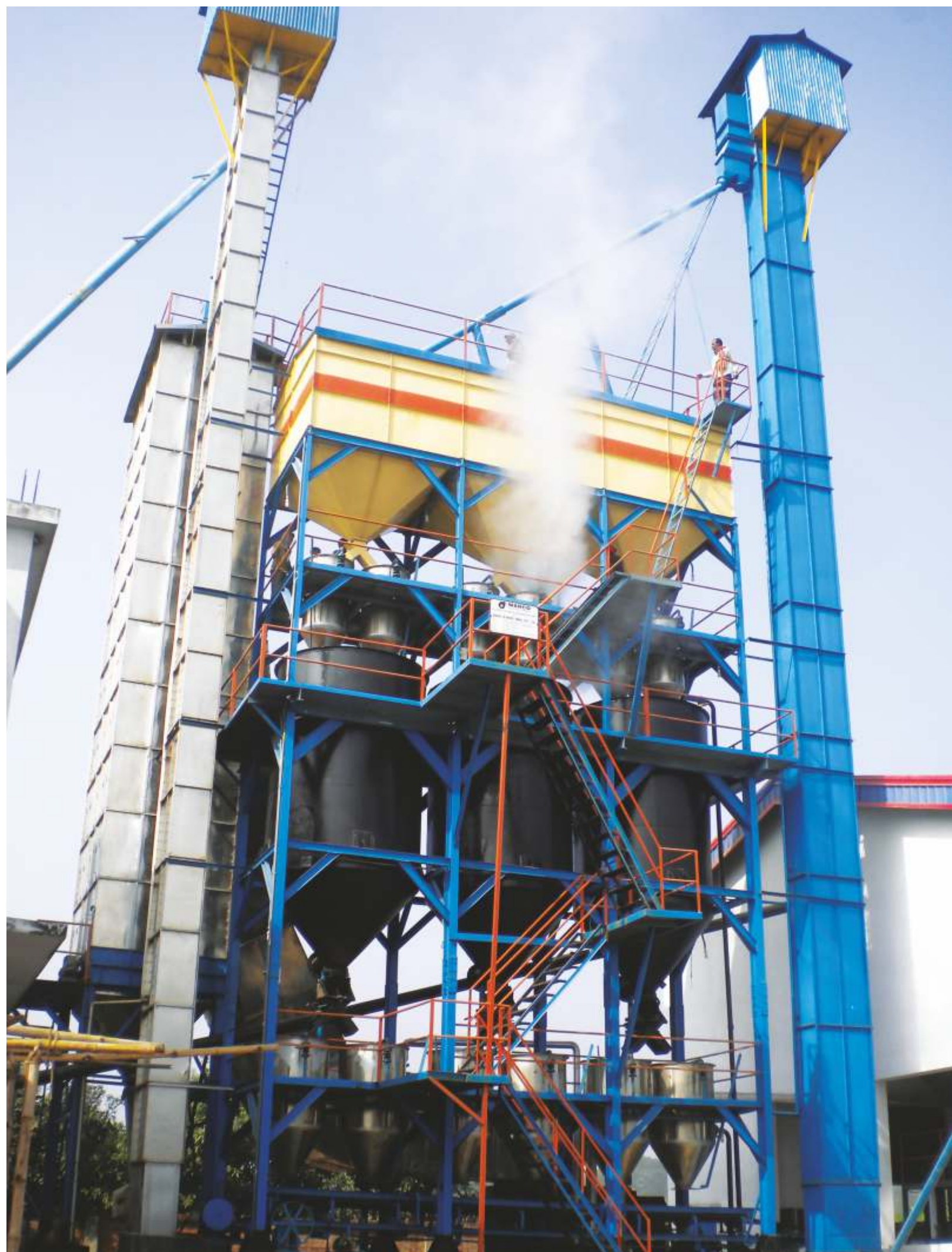
1 X 24 TON THREE STAGE PLANT
