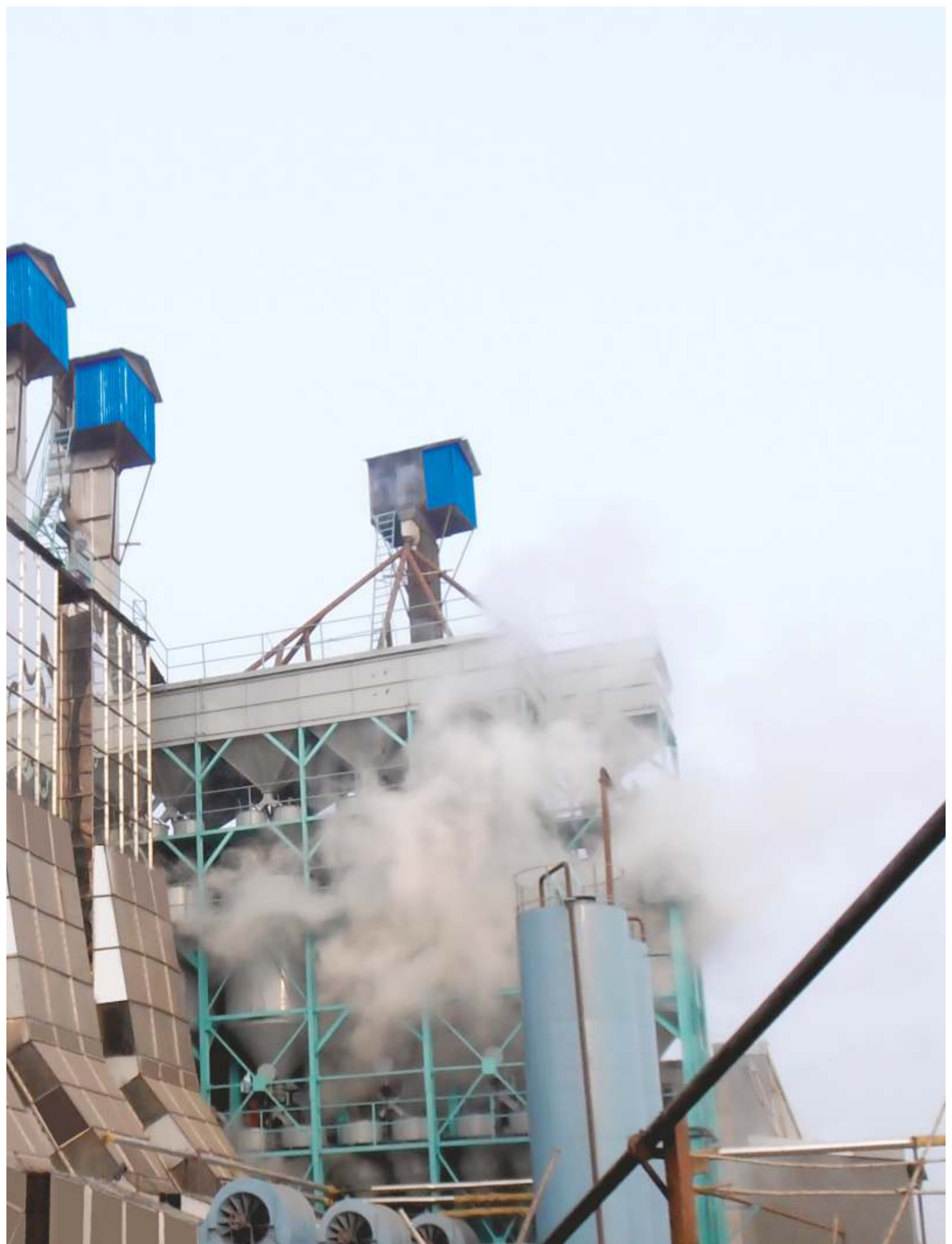
Parboiling Plant At Chapai Nawabganj , Bangladesh
